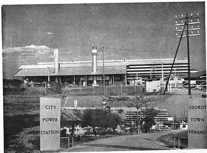
Penang Power Station (new 4th extension in foreground)
